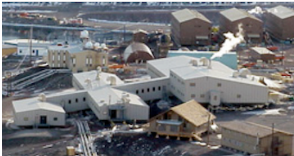
Albert P. Crary Science and Engineering Center, 1991
