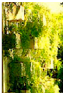
R: Living Wall installation, Baltimore, MD. This 110 sq ft (10 sq m) wall filters all the air for its 7,500 sq ft office building. Notice the ornamental character of some plants chosen
