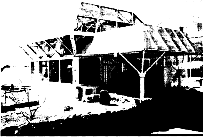
Fig. 4. The Biosphere II Test Module, which is 12,800 cu ft of volume in the biochamber. When the variable volume chamber is included, the total is about 17,000 cu ft. Experiments have been conducted in it since January 1987, and are ongoing, including human closed ecosystem work.
