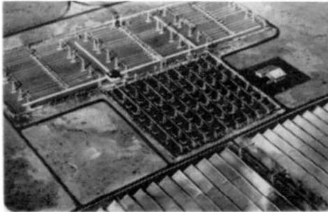
311 Inverters and standard power grid at the edge of the rectenna array over farmland.
