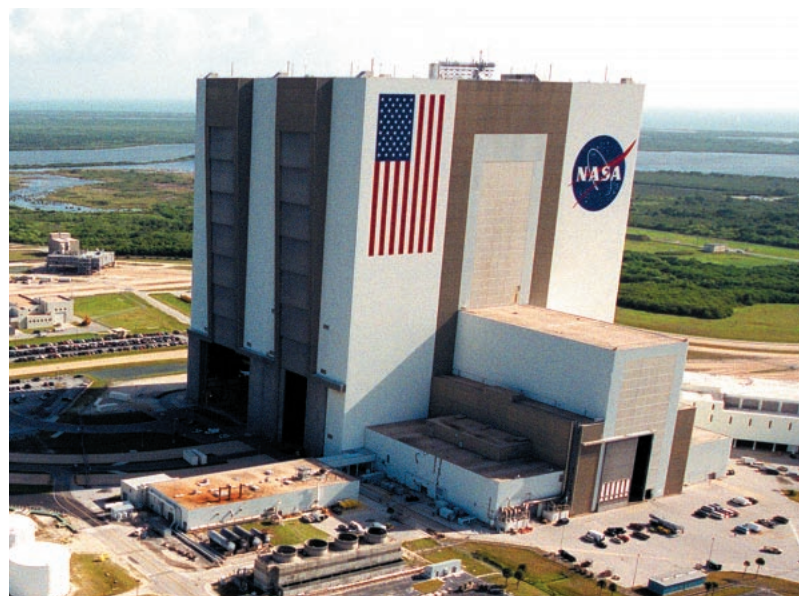
Kennedy Space Center's Vehicle Assembly Building.
